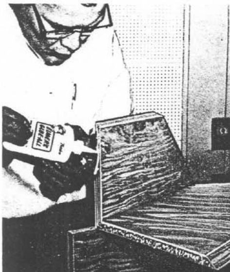
Fig. 24—Prime the joint surface with a thin coating, then put on a thick layer and assemble at once. Plastic glue will set in about thirty minutes.
