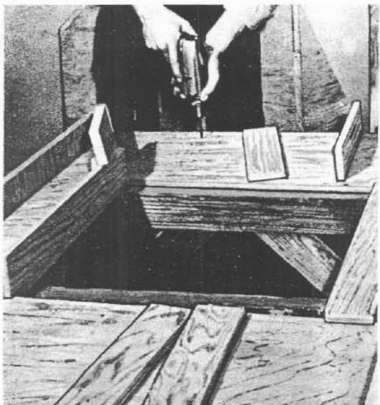
Fig. 15—Drilling for Assembly.
