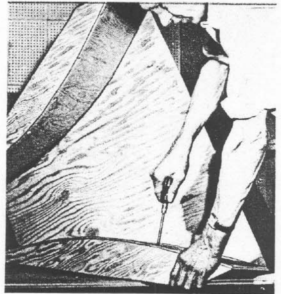
Fig. 12—Drawing the Joint Snug.
