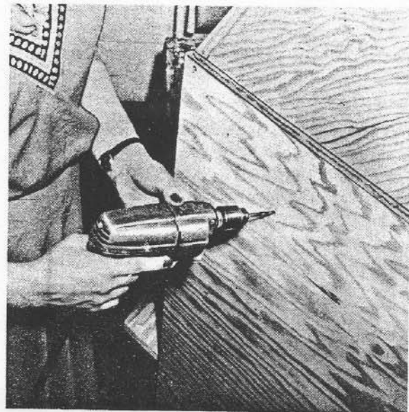
Fig. 23—Drilling for 10 and 11.
